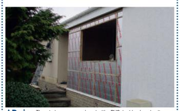
▲ During: The windows were replaced with uPVC double glazed units to enhance the home and give more windowsill space in the lounge. The Billingtons replaced old fashioned splay bays with box bays, installed with GRP gallow brackets to the underside and a feature tiled roof canopy which would continue across the home and match the new tiled roof.
