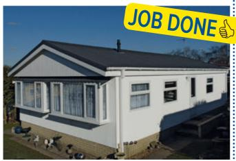
▲ After: New, maintenance free, uPVC fascia/barge boards with guttering were installed. This allowed Rapide to increase the pitch of the roof pre-formed gable ends with white uPVC open 'V' board cladding and trusses with lateral/ diagonal bracing where screw fixed into the original roof. Klober reinforced underlay and tanalised battens where then secured to the new roof carcass. Finally the granular lightweight tiles and trims were fitted.
