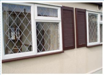
▲ **Before:** The original plywood texture coated outer walls were showing serious signs of decay, some of the boards had rotted and the drip bar had perished. The outer wall boards needed to be removed and the original wall structure would need to be checked over. After explaining and discussing the various wall renovation options available, the Billingtons decided to opt for the total non-maintenance, energy-efficient, thermally-enhanced wall renovation.
