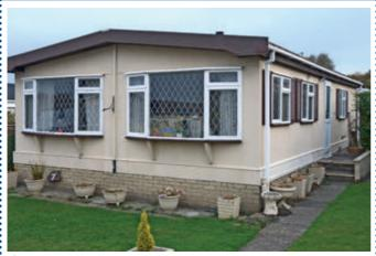
▲ Before: The roof covering was still the original Hyplon blanket and had perished over the years. Water ingress was evident so Rapide suggested to replace it with a new granulated lightweight pitched tiled roofing system. There was also evidence of rotting fascia/barge boards and the guttering was on its way out and leaking.
