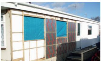
▲ During: The existing outer wall boards had to be removed and rotten timbers replaced from the existing wall structure. The wall thickness was doubled by screwing tanalised timbers onto the structure. Thermax PIR insulation board was fitted inside the new wall structure on top of the existing quilt insulation. Vinytherm uPVC cladding board was installed
