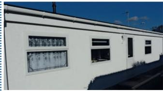
▲ After: Vinytherm has a unique integral cavity which creates a continuous air circulation between the additional insulation/structure and the outer wall surface. This results in a maintenance-free outer wall finish and an enhanced thermally efficient wall structure keeping the home free from condensation and rot while being warmer in the winter and cooler in the summer.
