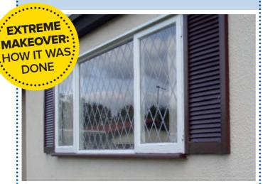
▲ **Before:** All the original single glazed wooden windows were showing signs of decay or rot. The doors had been replaced with uPVC but these had been poorly fitted and were made for a bricks and mortar home. They needed to be replaced with uPVC double glazed units which would be fabricated with an odd leg outer frame, specifically for park
