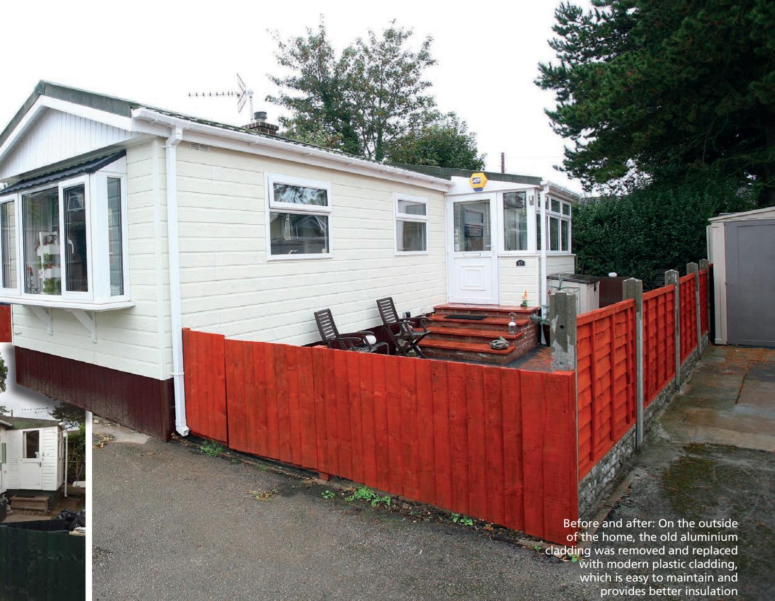
Before and after: On the outside of the home, the old aluminium cladding was removed and replaced with modern plastic cladding, which is easy to maintain and provides better insulation
